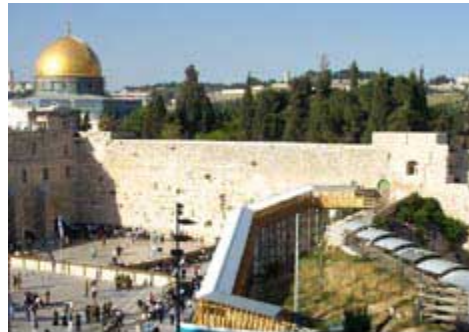
The new temporary ramp (with white roof), and the old broken ramp at the right.
